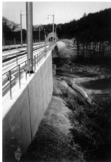
Figure 2. GRS-RW with a FHR facing constructed to support bullet train tracks (Hokuriku Shinkansen) west of Karuizawa (Location 50, Figure 3): (a) typical cross section (gravel-filled gabions are not shown); (b) wall under construction; (c) completed wall.
